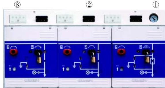
① Barometer ② Indicator ③ Fault indicator
